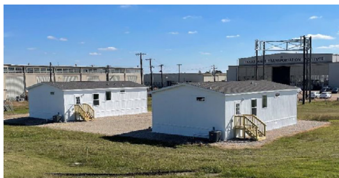
Photo 1. The Texas A&M Smart and Connected Homes Testbed (TAM-SCHT)
